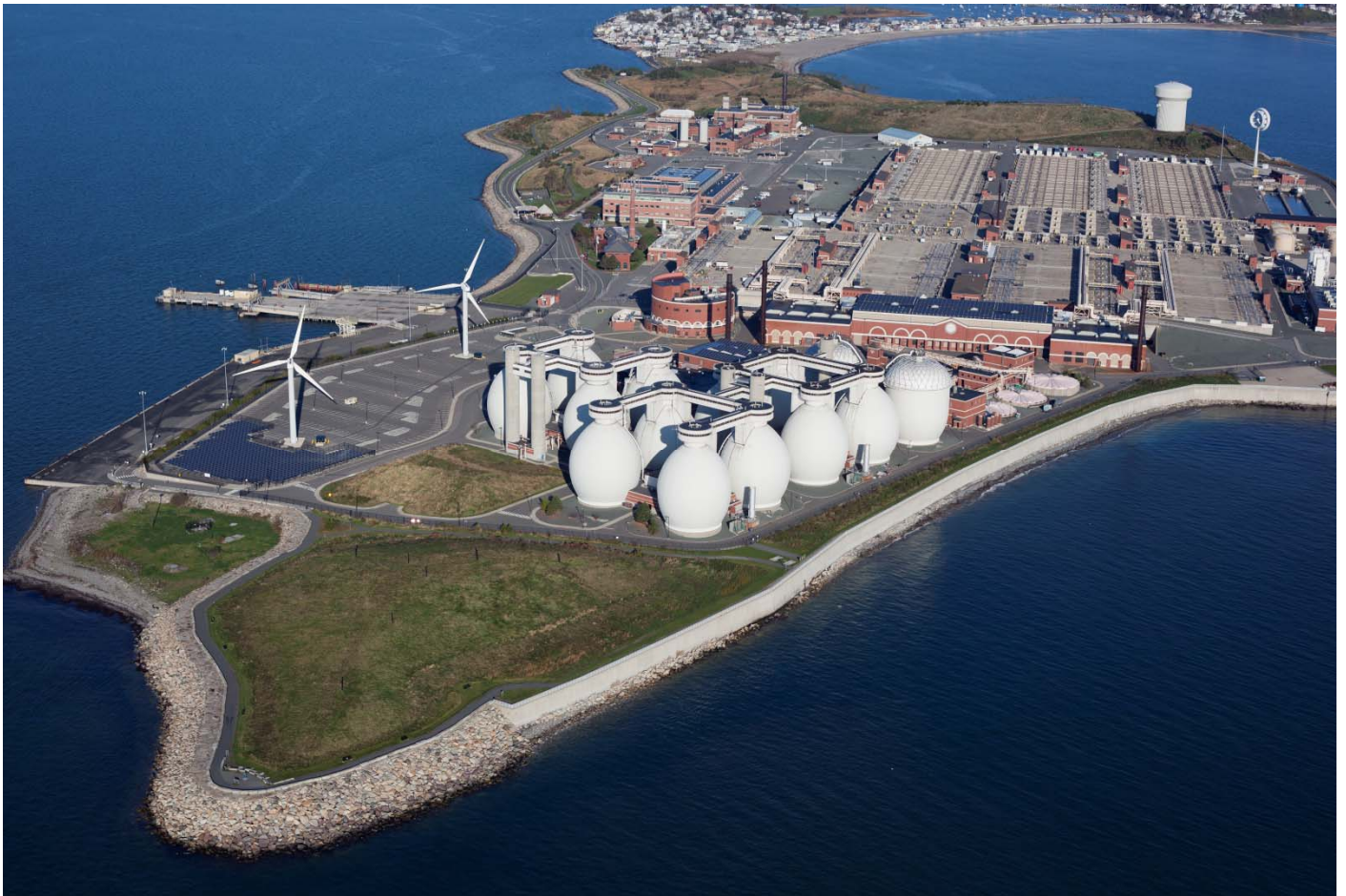
Deer Island Wastewater Treatment Plan
